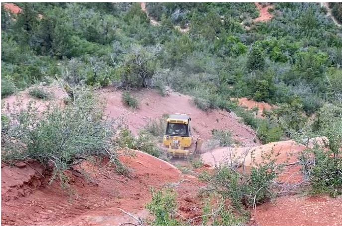
ROADWORK UNDERWAY THROUGH THE RED ROCK
